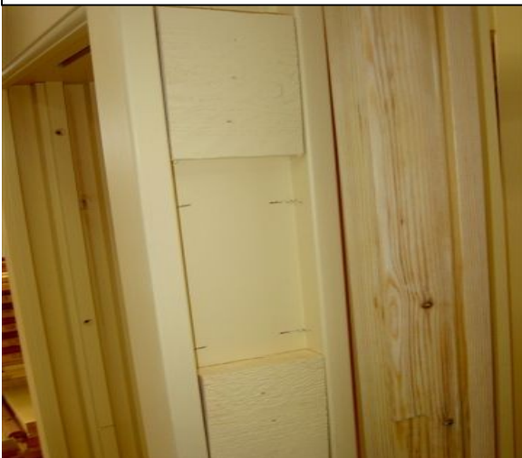
Using CF's to secure Box Window
